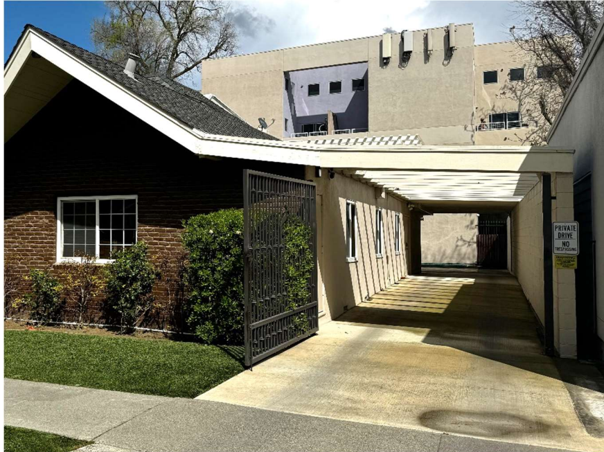
Side (south) façade, view facing northeast. Source: ESA, 2024.
