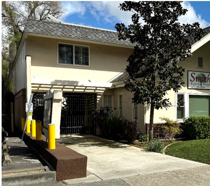
Side (north) façade, view facing southeast. Source: ESA, 2024.
