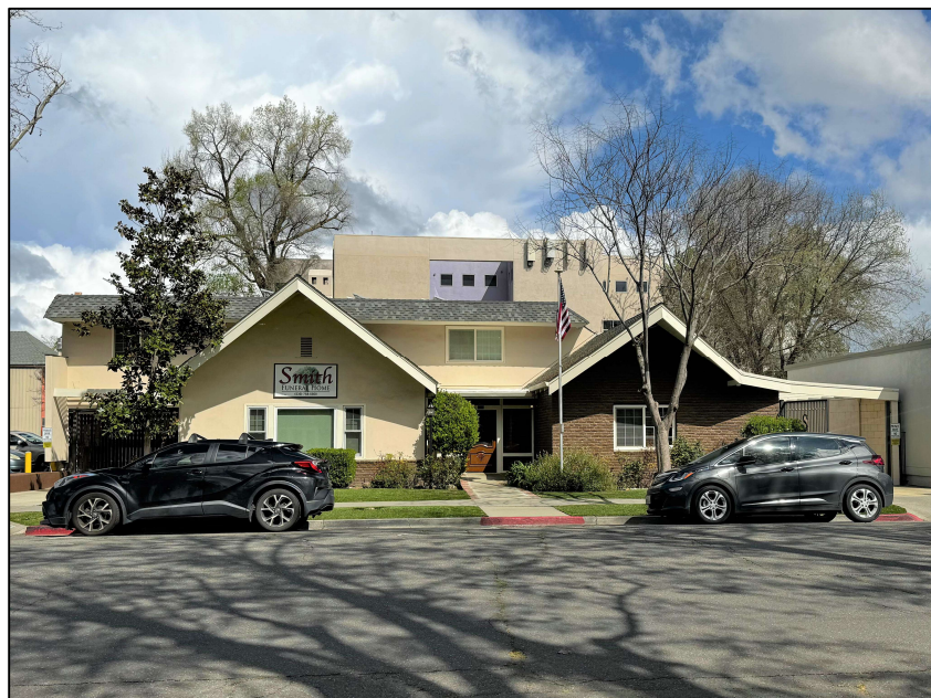
P5b. Description of Photo: Primary (west) façade, view facing east. March 30, 2024.
